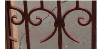
local wrought iron details
