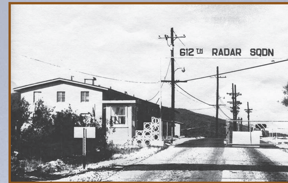
Main gate of cantonment with bachelor officer's quarters at left, ca. 1962.
