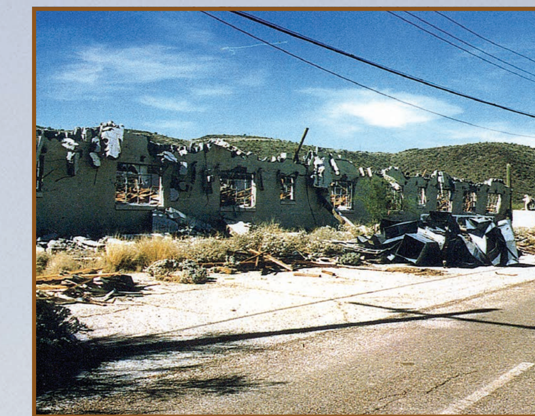
Demolition of administration building, 1995.
